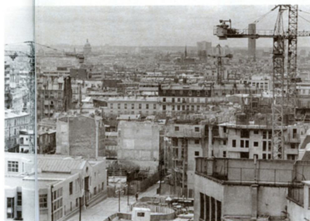
Belleville. Looking south to the Tour Montparnasse.
