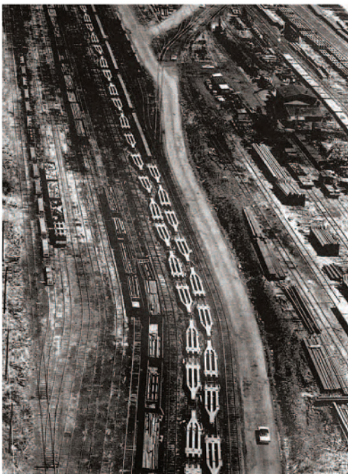
WTC spandrels being transported to the construction site.
